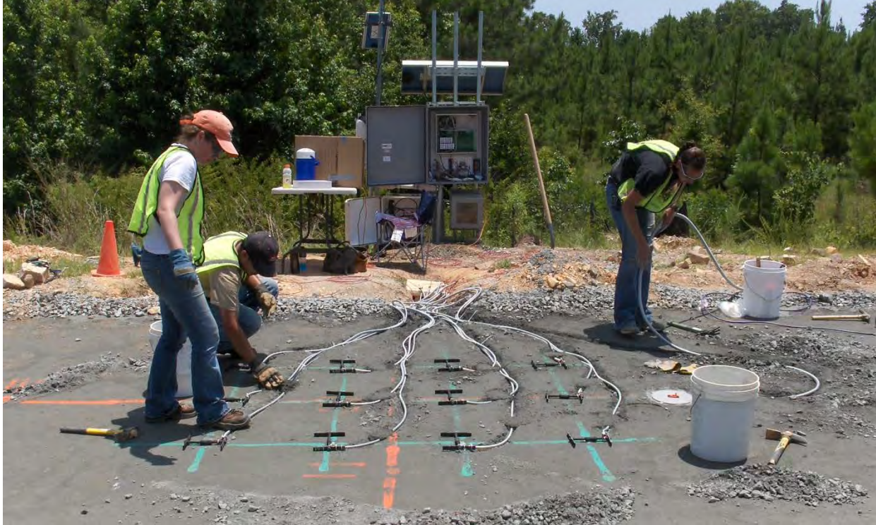
Figure 1.2 Installation of Strain Gauges and a Pressure Plate Before Placing the Asphalt Base Course
