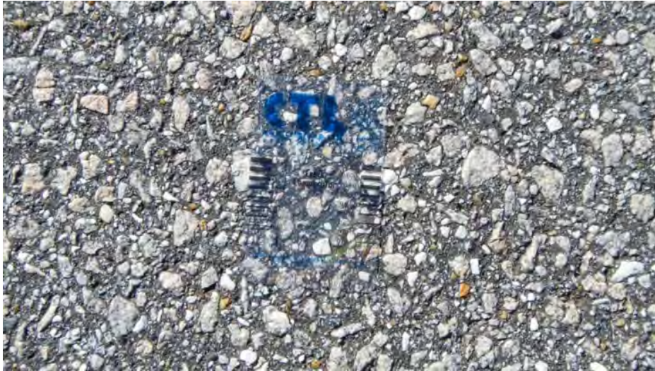
Figure 3.5 Close-up Photograph of Section W5 Showing Texture and Hairline Crack Just Below the Scale
