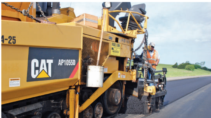
Original HiMA pavement placed in 2012 by Haskell Lemon Construction Co.
