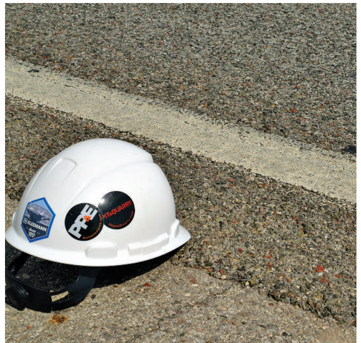
“Popcorn” thin open-graded friction course performs on I-40 HiMA pavement.
